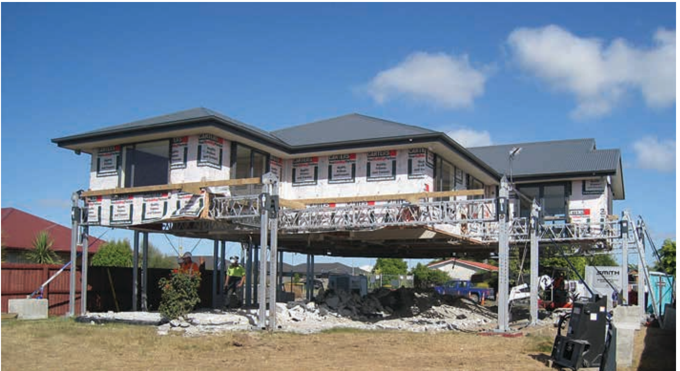
A house being lifted with Smith Cranes' synchronised jacking plant
